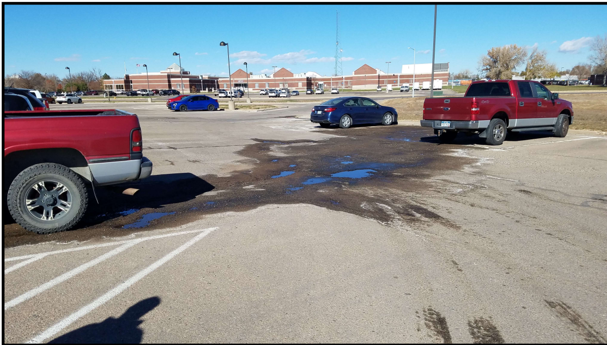
East Parking Lot Low Area
