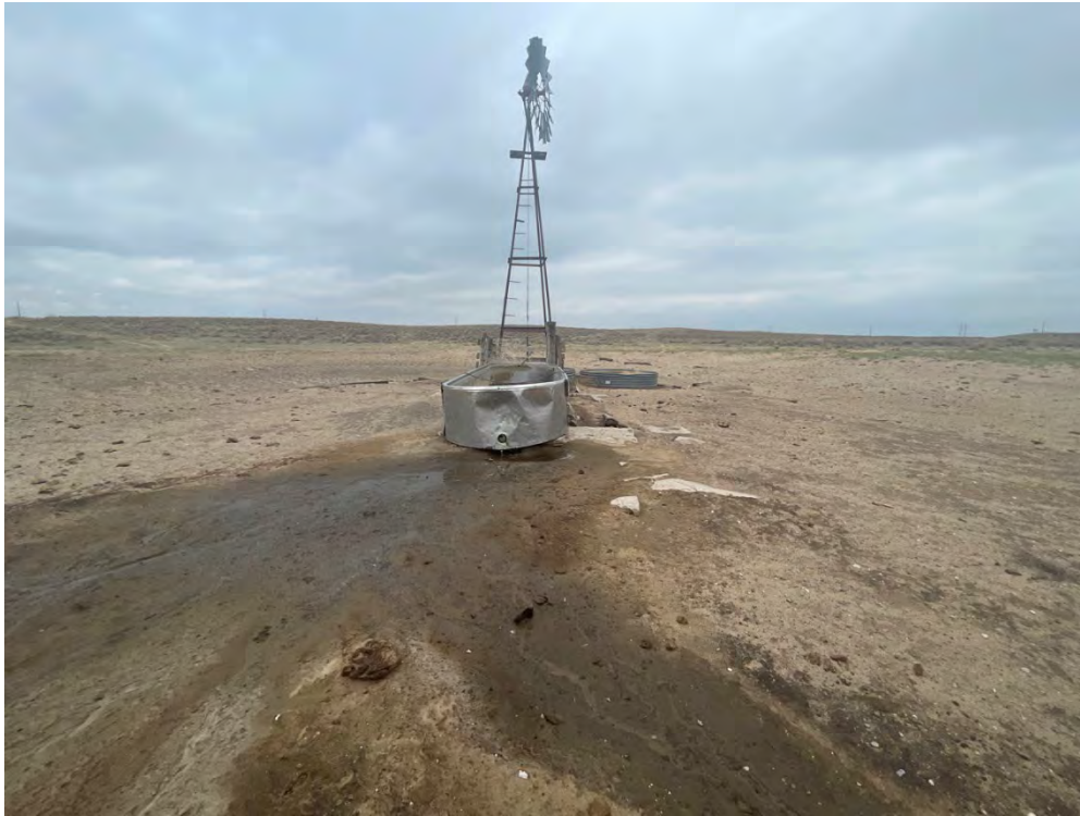
Photo 7: Typical aboveground water storage tank for cattle. View is looking north.
