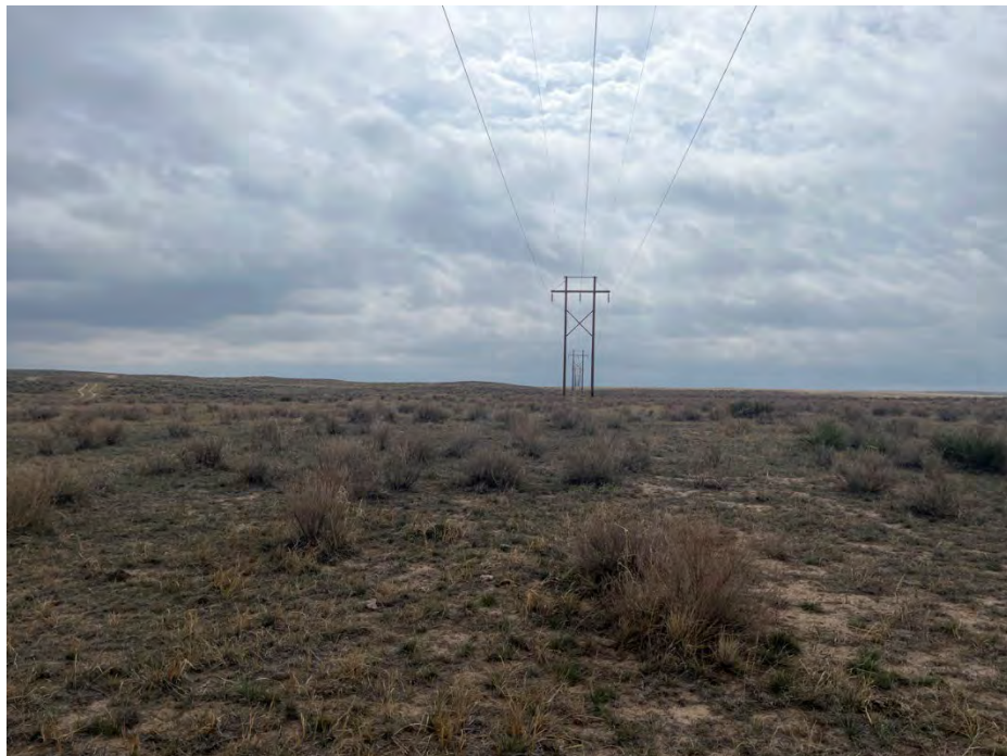
Photo 14: Existing transmission line located within the Project Area. View is looking southeast.
